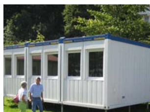
Office container buildings
