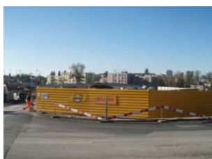
Construction site fences
