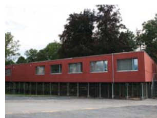
Container systems on piers
